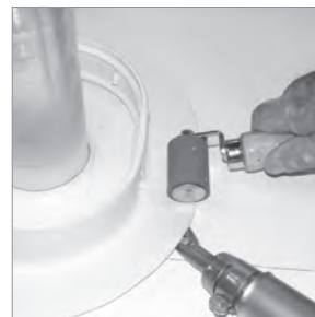
3. Heat weld vertical &amp; horizontal seams first
