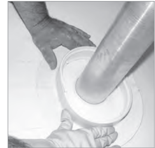
2. Ensure proper fit of 2 piece PVC Molded Sealant Pocket
